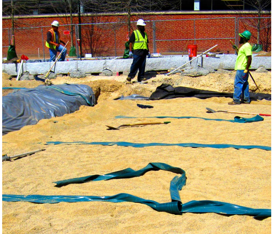
Figure 23. Sand Storage Bed Below the Lawn (Credit: Andropogon Associates)
