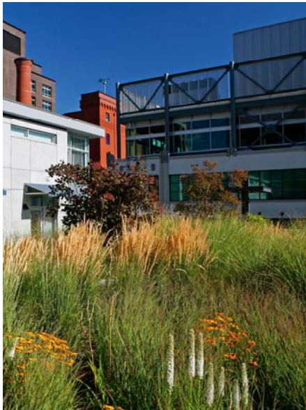
Figure 17. Vegetation on an intensive roof. Courtesy Green Roofs for Healthy Cities and Walker Macy Landscape Architects
