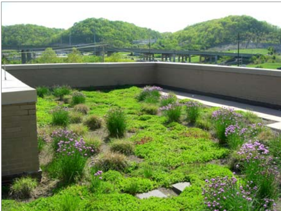
Figure 16. Vegetation on an extensive roof. Courtesy Green Roofs for Healthy Cities and Sanitation District No. 1, Wright, Kentucky
