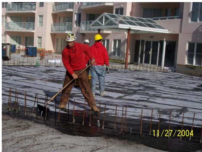
Figure 13. Hot-applied rubberized asphalt. Courtesy Jeffrey Bruce, FASLA
