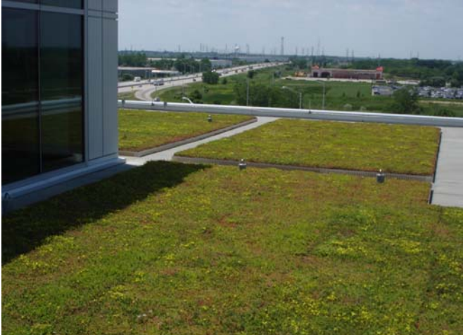
Figure 18. Pre-grown sedums on an extensive roof. Courtesy Green Roofs for Healthy Cities and Intrinsic Landscaping, Inc.
