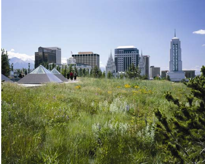
Figure 2. The Church of Jesus Christ of Latter-day Saints Convention Centre, Salt Lake City, Utah Semi-intensive green roof combining areas with growing medium of greater and less than 6 inches Source: Olin Partnership
