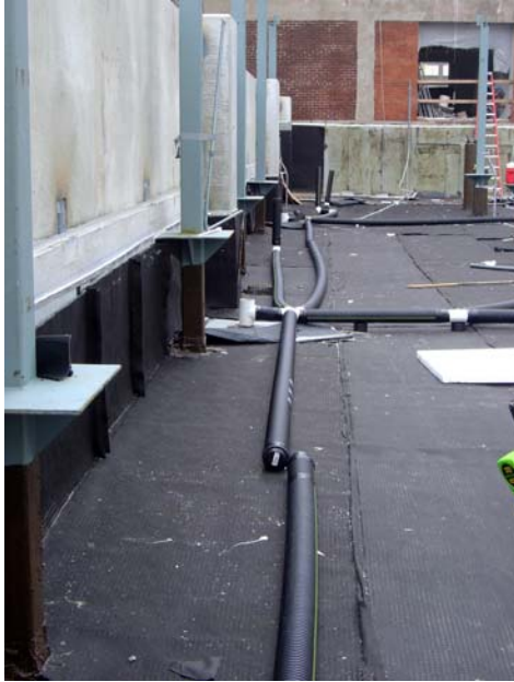
Figure 14. Drainage pipe on membrane. Courtesy Jeffrey Bruce, FASLA
