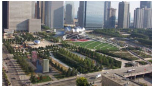
Figure 5. Millennium Park. Courtesy Green Roofs for Healthy Cities and Terry Guen Design Associates, Inc.
