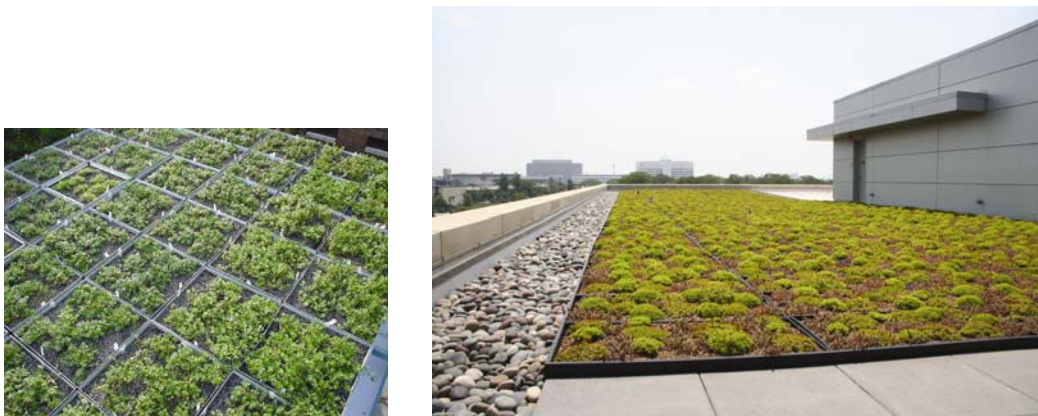
Figure 4. Modular components. Source: Green Roof Blocks (left, smaller image); Greengrid (right, larger image)
