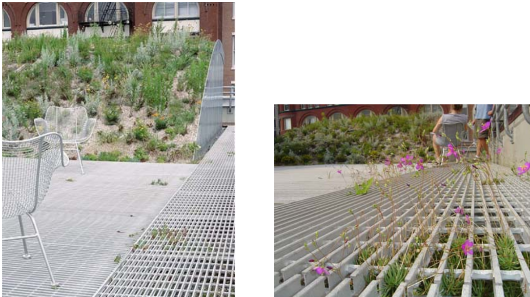
Figure 17. Two illustrations of grating used as a walking surface over planted sedums. Courtesy MVVA
