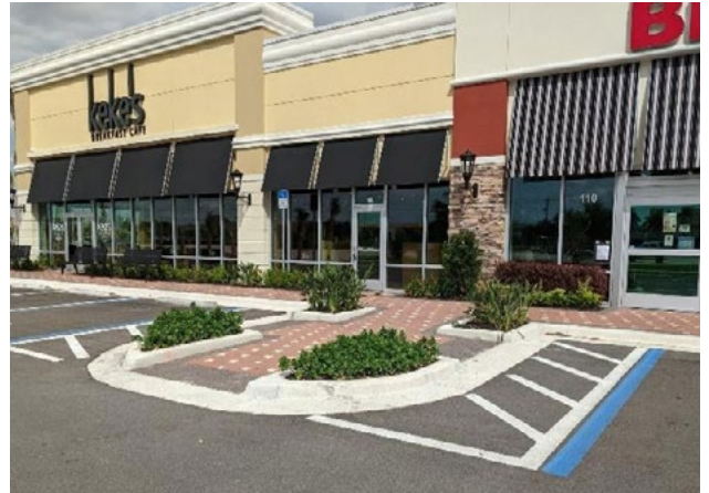
Figure 8. Innovative yet conforming dual ADA curb ramps
