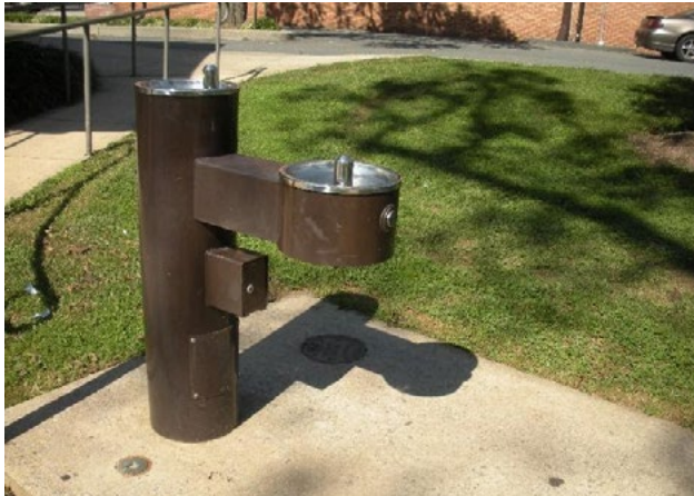
Figure 13. Accessible dual height drinking fountain
