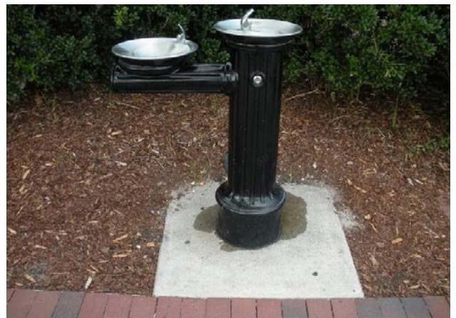
Figure 54. Water fountain lack of accessible excessive surfaced clear ground area. Applicable ADA 2010 Code Standards: 602.2 (whole section)
