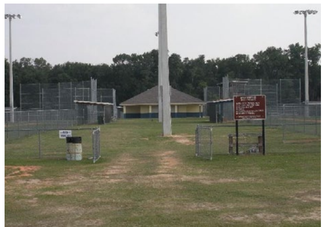
Figure 36. Lack of accessible route to sports fields, support facilities, player and spectator seating. Applicable ADA 2010 Code Standards: 206.2.2, 402 (whole section)
