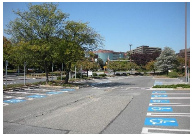
Figure 24. No access aisles; accessible route behind cars required. Applicable ADA 2010 Code Standards: 402 (whole section), 502 (whole section)
