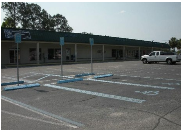
Figure 29. Nonconforming signage; lack of access aisles; ADA spaces not dispersed among shops or closest parking to building entrances. Applicable ADA 2010 Code Standards: 208.3, 502 (whole section)
