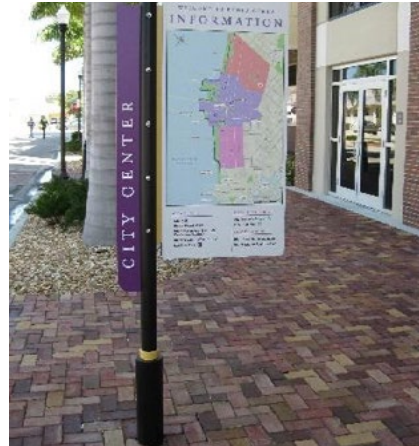
Figure 26. Sign creates protrusion into pedestrian travel way and no tactile elements. Applicable ADA 2010 Code Standards: 307.0, 403.5
