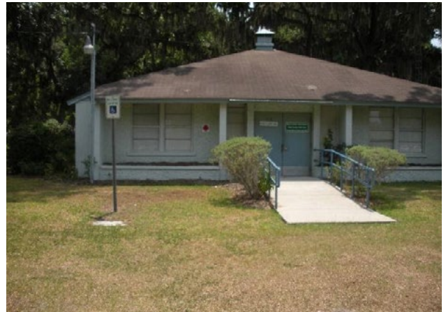
Figure 46. No accessible parking space; no accessible route; no handrail extensions. Applicable ADA 2010 Code Standards: 206.1-206.2.2, 405 (whole section), 502, 505.10
