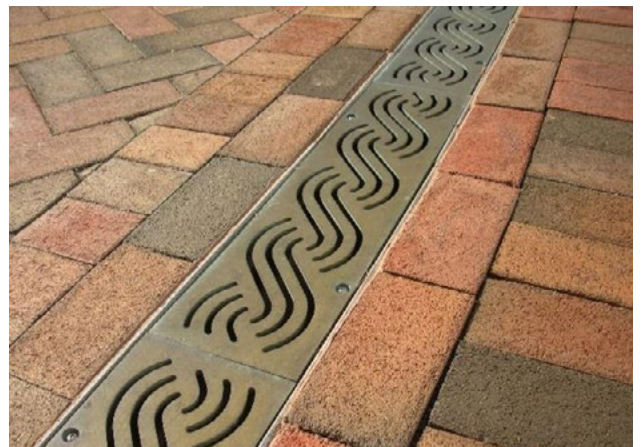
Figure 12. Decorative ADA conforming drainage grate in accessible route
