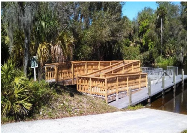
Figure 5. Accessible route to boat ramp loading/unloading dock
