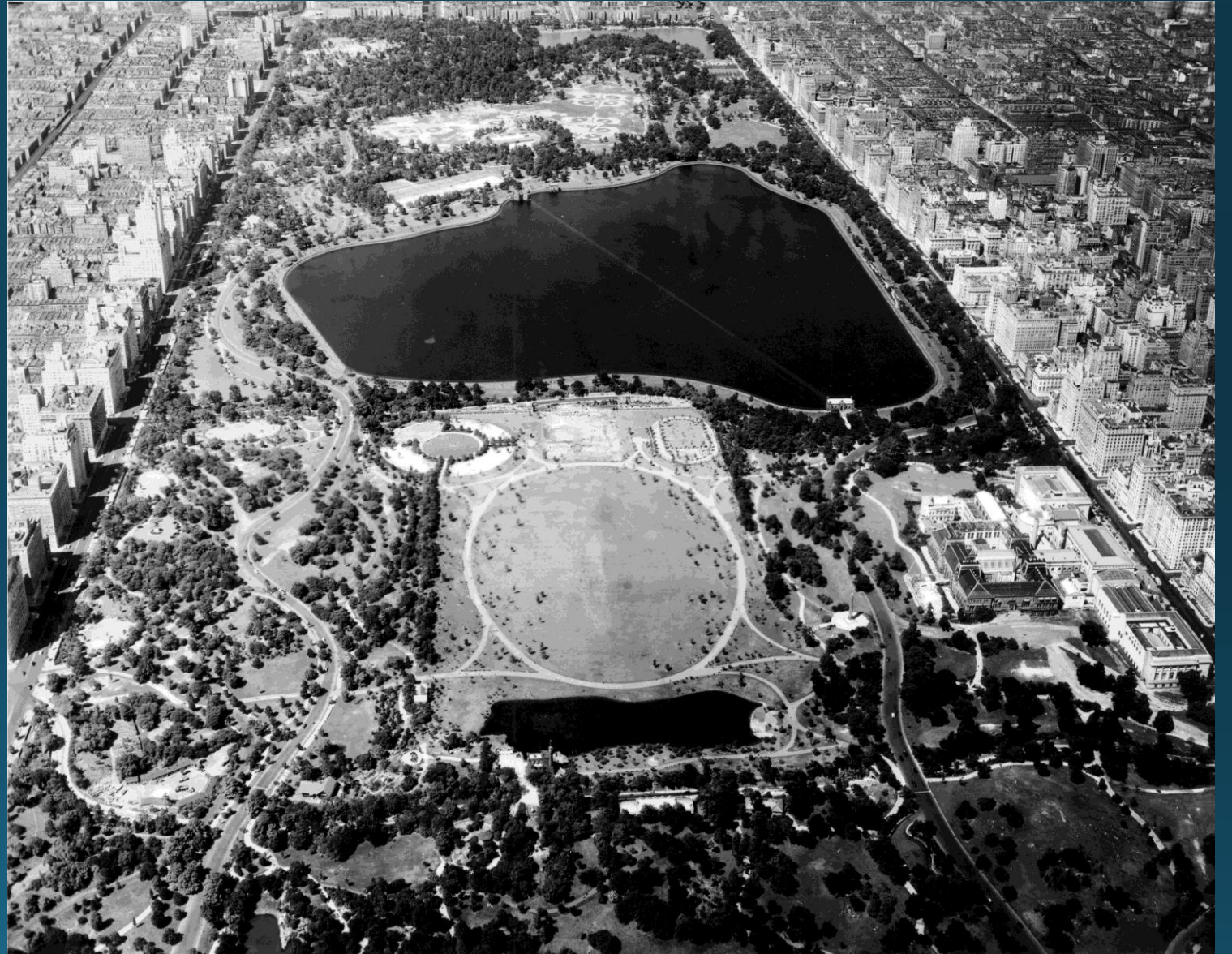
Aerial 79th Street to 110th Street, View North 6-24-1938
