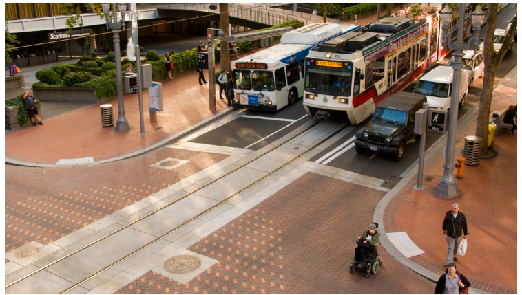
Landscape architects plan and design transportation corridors that consider all users of the roadway—cars, cyclists, pedestrians, mass transit riders, and more. Photo: Bruce Forster Photography, Inc.
