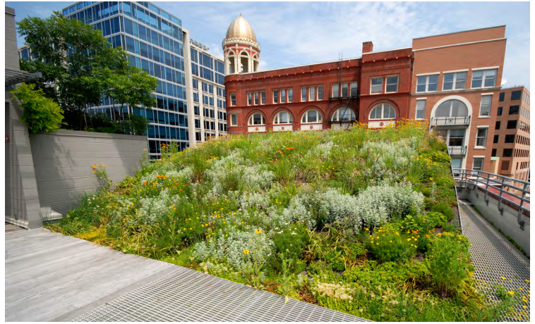
ASLA headquarters' green roof is one example of how landscape architects help reduce stormwater runoff while also conserving energy and improving air quality. Photo: ASLA
