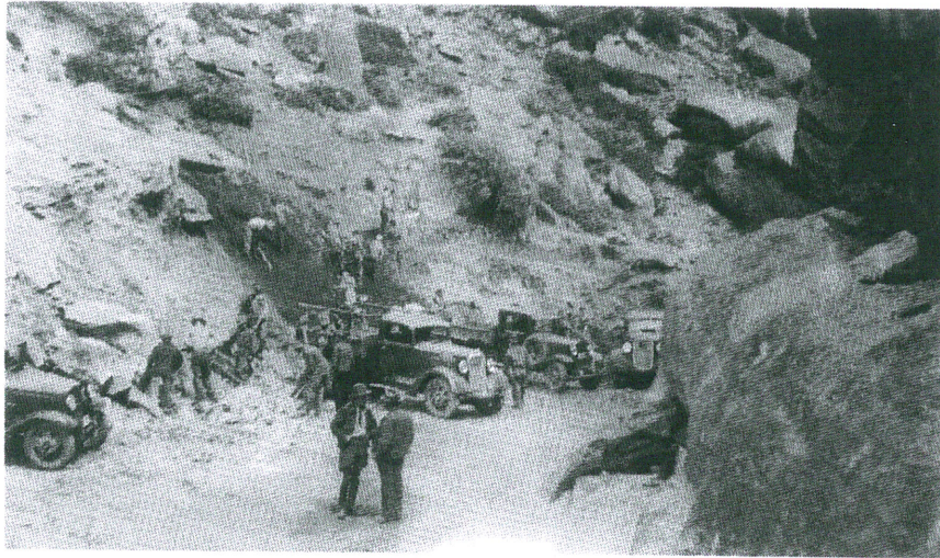
FIGURE 13. May–July 1936. Before the theatre was designed, enrollees built the stage, first cutting and filling the area around stage rock by hand (NA).
