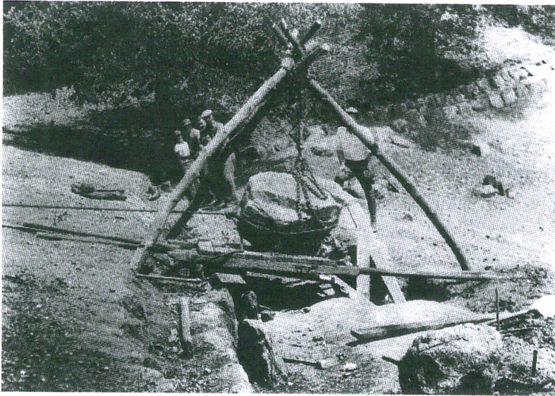
FIGURE 39. 1934. Initially, tripods of onsite timber were utilised to move the 1000–4000 pound stones. Note the NPS foremen in his regulation hat and jodhpurs (NA).
