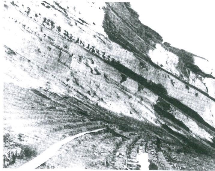
FIGURE 18. Mid-1937 Rather than maintain a traditional level elevation along the seating rows, Hoyt and Morse sloped the entire theatre 3.33% from north to south in line with the rock strata underlying the entire landscape (NA).
