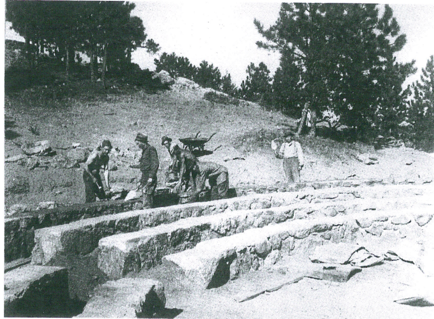
FIGURE 5. Enrollees mortar local stone at Flagstaff (NA).
