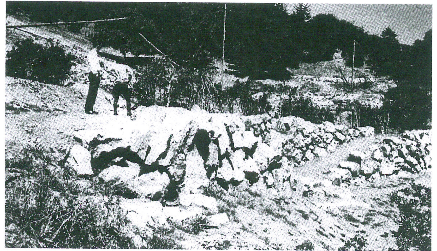
FIGURE 37. Stone retaining walls supported the 12 feet of fill in the ravine that once crossed the stage. These walls also allowed actors to move from stage left to stage right without being seen (MHS).
