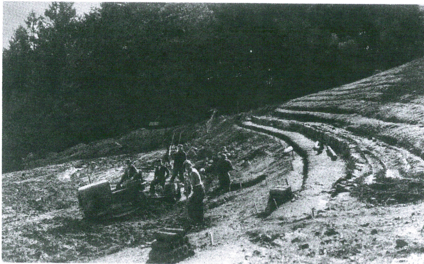
FIGURE 35. In April 1934, construction began. With the only earthmoving equipment ever used on the site, enrollees re-graded the stage, installed drainage and water supply lines and began the rough terracing of the lower seats, following the alignment of the existing 1929 row (MVPL).
