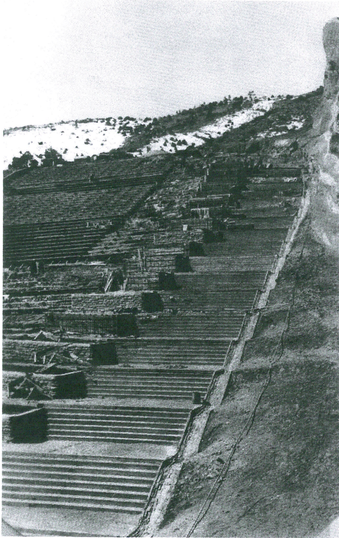
FIGURE 22. 1938. To mesh the theatre and the newly revealed ledge, enrollees did not pour the seats all the way out to the northern edge until the north stair and planters were built bugging the exposed ledge of Creation Rock. Seating was built from the middle (left to right in the photograph) and the stair out from the rock wall (right to left) to eventually meet. The stair planters were similarly test built to fit (DPL).
