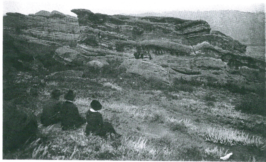
FIGURE 9. The topography and the surrounding rock formations carried sound from stage rock to the top of the site 1000 feet away. During construction, workers monitored the acoustics by spinning a coin on stage and checking if its fall could be heard at the top of the theatre (DPL).
