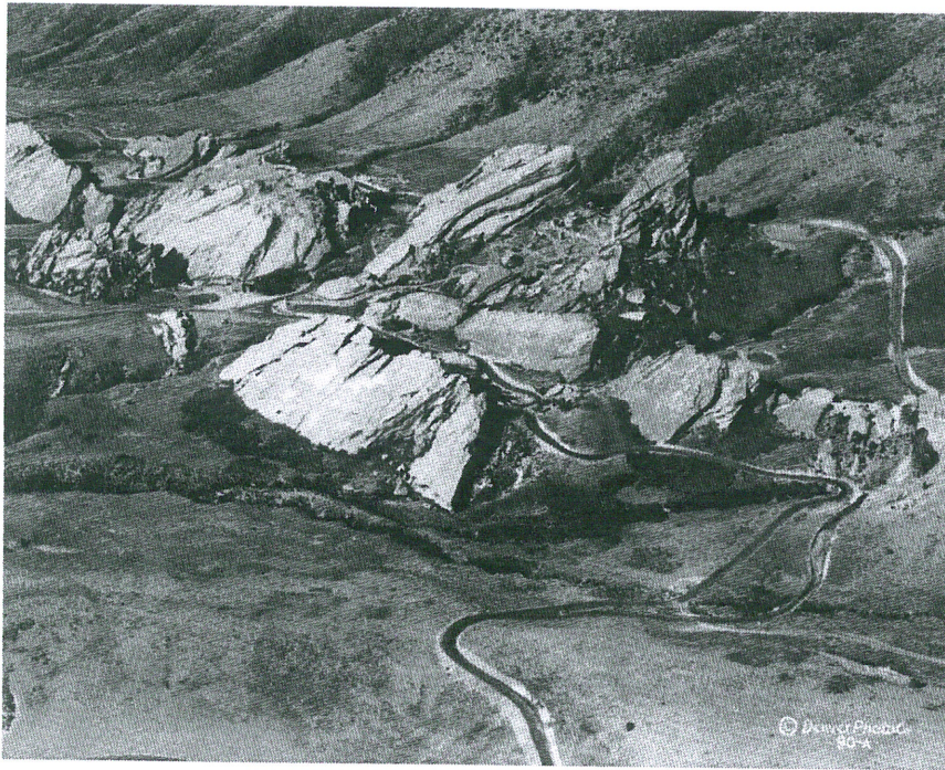
FIGURE IO. 1929. An aerial view shows the scenic road built to the site to boost the idea of constructing an amphitheatre. Compare this view with the post-construction aerial, figure 26 (DPL).
