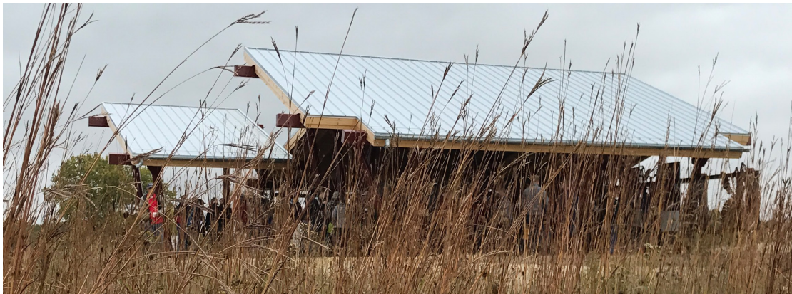
Nachusa Visitor Use Center, construction almost completed, October 2017.
