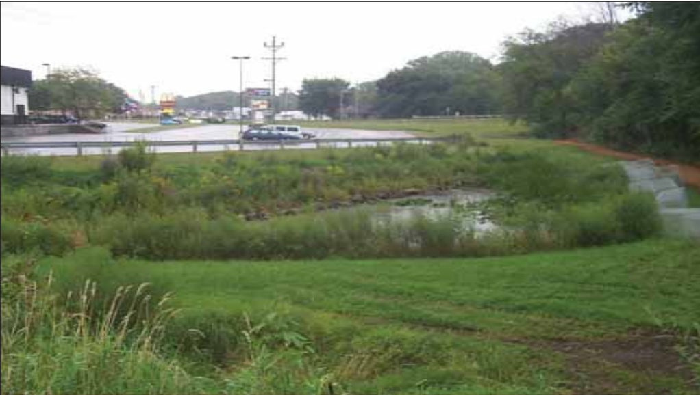
Naturalized detention ponds can be used to store large volumes of stormwater runoff, while filtering contaminants out of the water and allowing for infiltration into the ground-water table.
