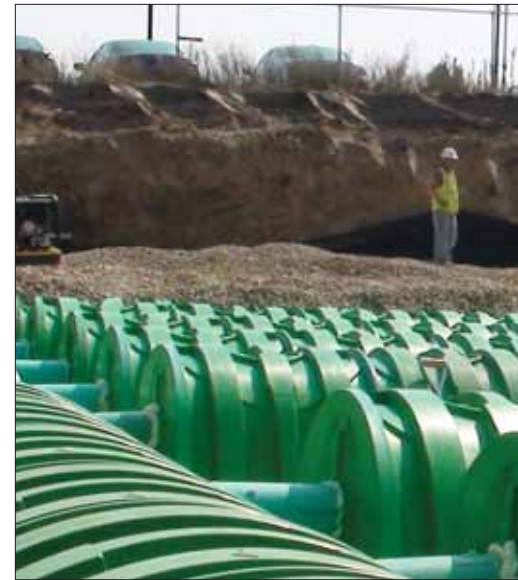
Subsurface detention tanks can assume a variety of shapes and sizes. These structural arches are intended to be used beneath parking lots or other load bearing surfaces.
