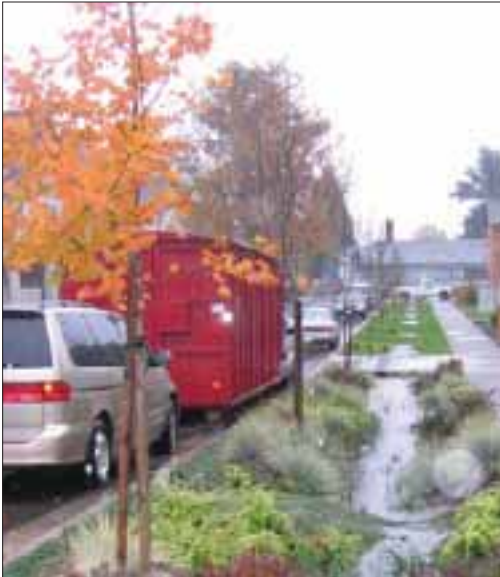
Vegetated swales assist in conveying stormwater runoff downstream, while helping to filter contaminants and allow for absorption by plants and soils.
