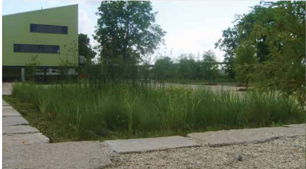
Rain gardens can take many shapes and sizes, and can be designed to function in a variety of ways. This rain garden in the Make It Right project area utilizes native plant species and is bordered by reclaimed concrete, helping to reduce minor flooding in the immediate vicinity. (photograph by Make It Right)
