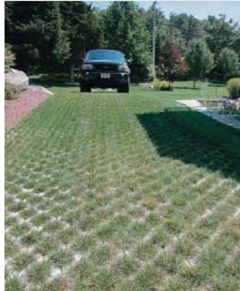
A driveway utilizing open-cell pavers planted with grass. Open-cell pavers allow stormwater to infiltrate into the void spaces, while still providing a durable driving surface in low traffic situations such as driveways.
