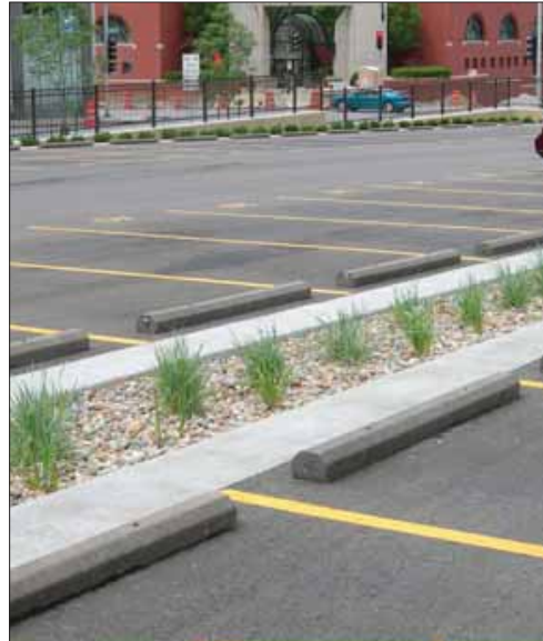
Vegetated swales can also act to intercept sheet flow from surfaces such as parking lots, helping to reduce runoff and filter contaminants.
